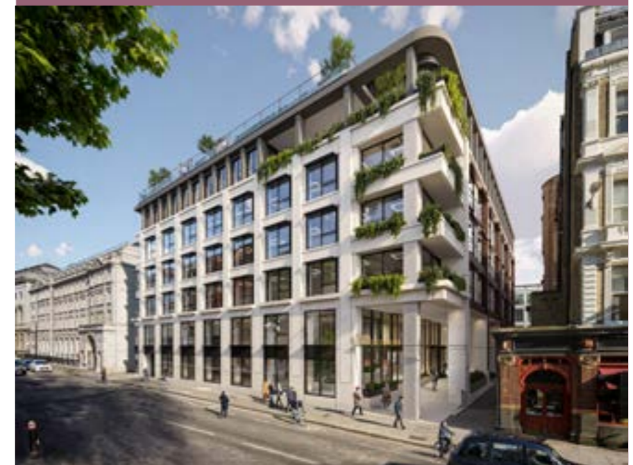
Giltspur Street facade showing extensive greening. Source: Design and Access Statement.
