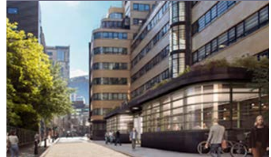
Visual illustrating the new steel Crittal windows to match original style. Source: Design and Access Statement.
